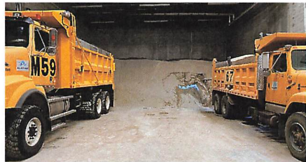
Figure 6: Sand storage building at ALB
