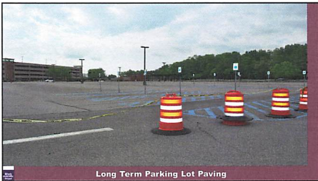
Long Term Parking Lot Paving
