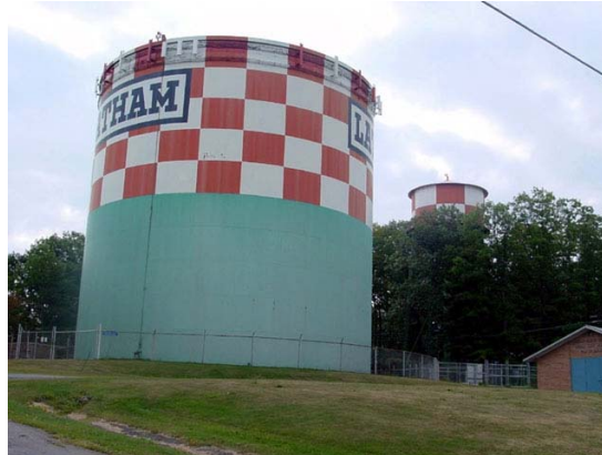
Latham Water Towers to be replaced
